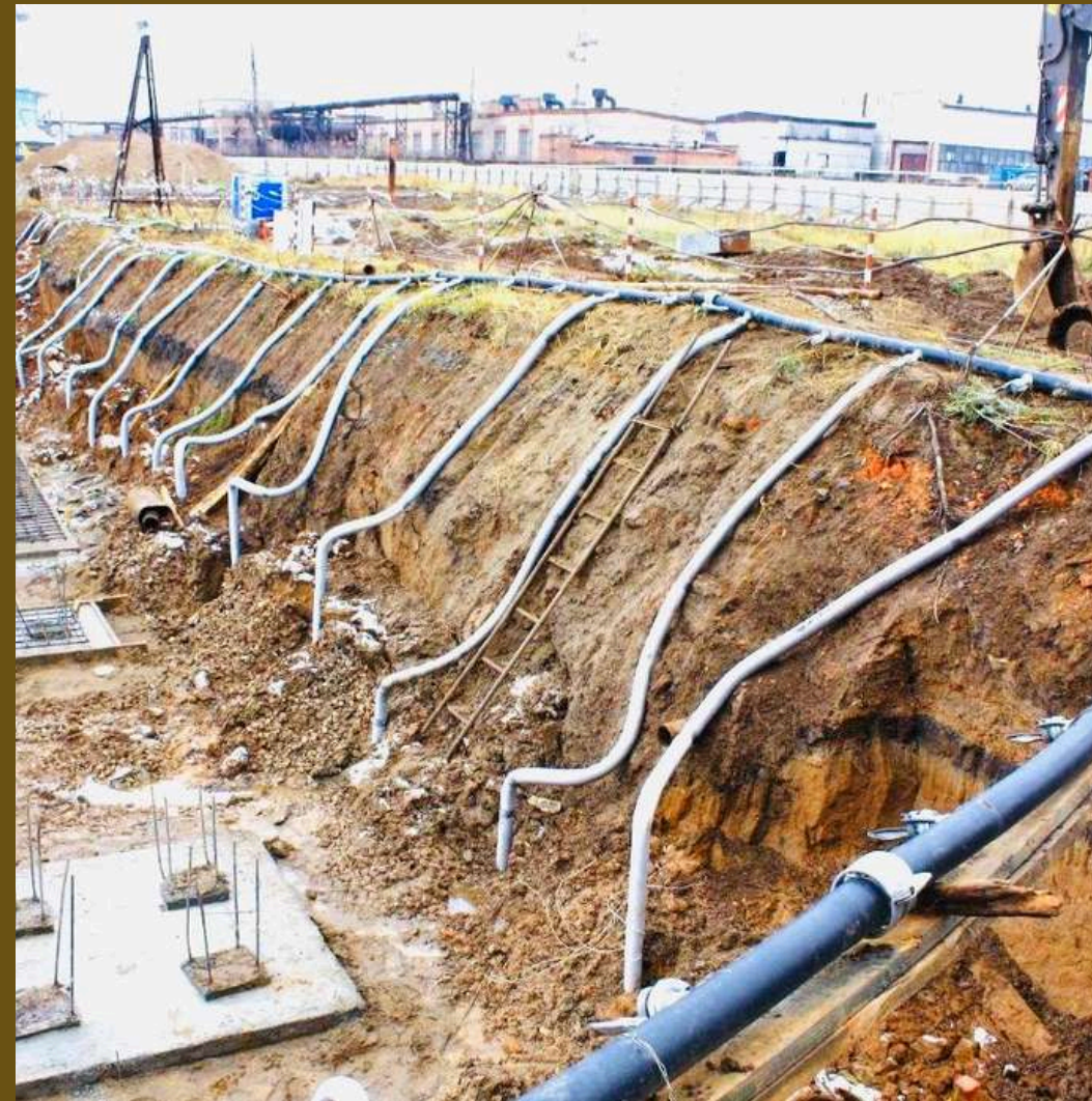
Wellpoint Design Installation & Commissioning
