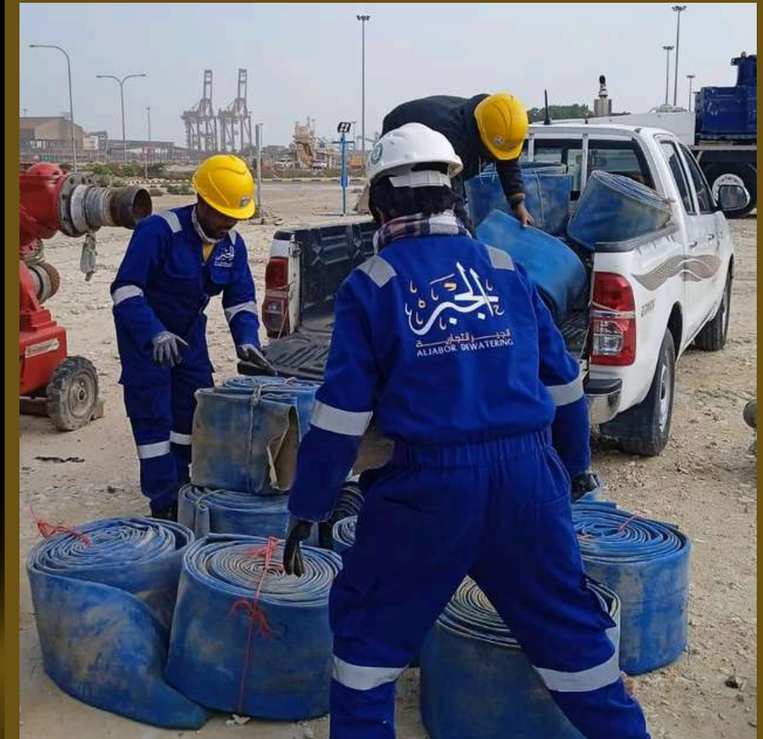
Pump Repairs Pump Maintenance
